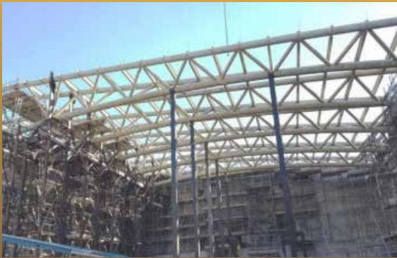
DUBAI – MORJAN project STEEL STRUCTURE
