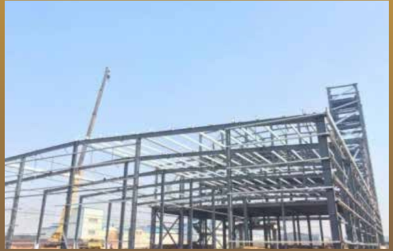
DUBAI store project STEEL STRUCTURE
