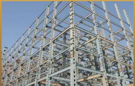
DUBAI – MORJAN project STEEL STRUCTURE
