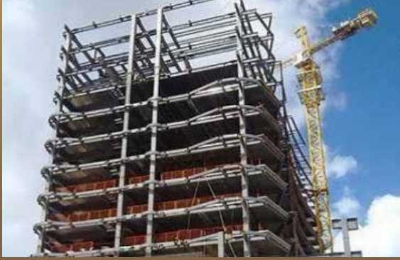
DUBAI – MANARA project STEEL STRUCTURE
